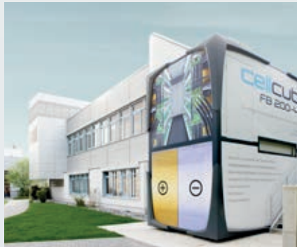
Energy solutions Park, Bielefeld, Germany
