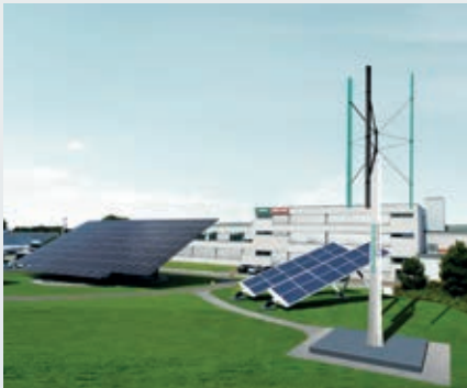
Energy solutions Park, Bielefeld, Germany
